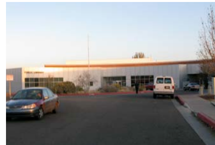
Alamosa Community Center, NM
